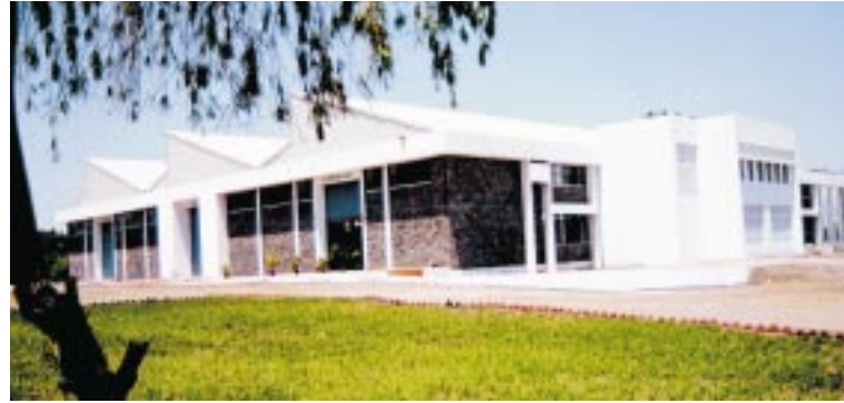
The Ahmednagar factory - manufacturing DC Motors
